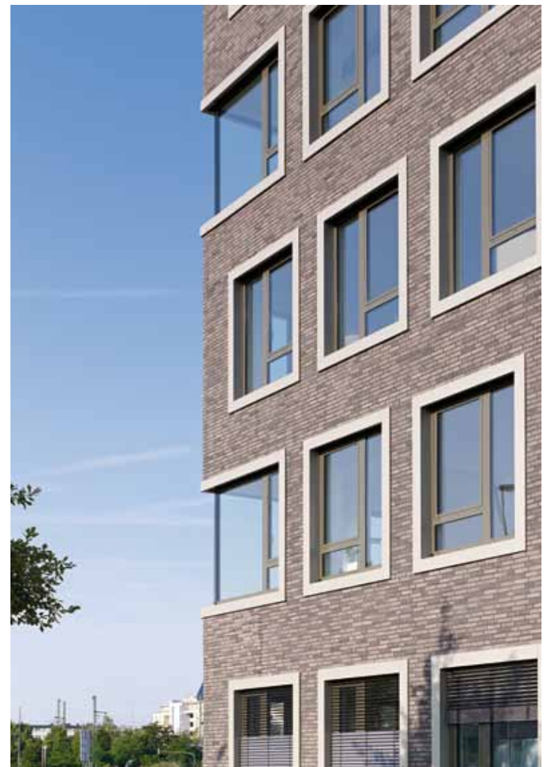
The facade was created on EIFS using 2,200 m 2 of thin format clinker brick slips, 21,000 corner pieces and 400 camber angle slips.
