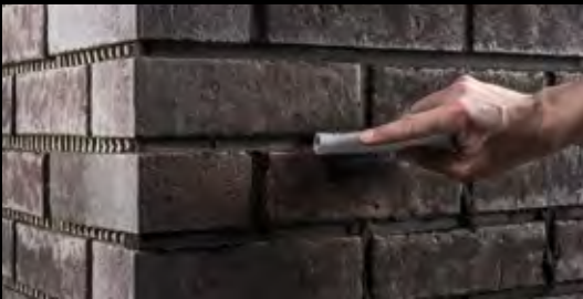
Jointing with a trowel allows you to create different looks.
