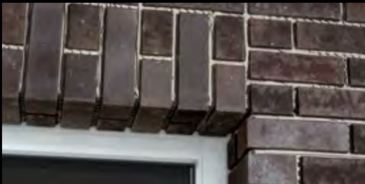
Window lintel perfectly replicated with angles.
