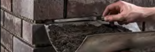
Grouting using pointing trowel and metal float along the horizontal.
